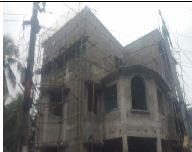
Construction work of Handicraft Training Centre at Baulagadia, Balasore (Under Progress)
