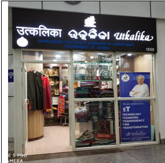
Renovation of Utkalika Branch at Terminal-1 of Biju Patnaik International Airport
